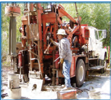
Percussion drill rig.
