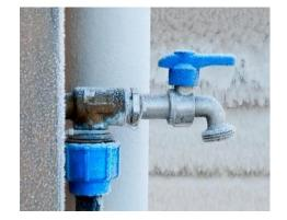
If your home has an outside faucet or spigot, there may be a shutoff valve somewhere inside of your home. Turn off the water supply to this faucet for the duration of the winter. First, close the shutoff valve then open the outside faucet to drain the remaining water from the pipe. This will protect the pipes that lead to the outdoors from freezing. If you do not have a shutoff valve, consider having one installed.
